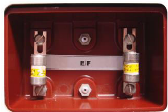
Fuse dimensions: Length 57mm x Diameter 13mm
